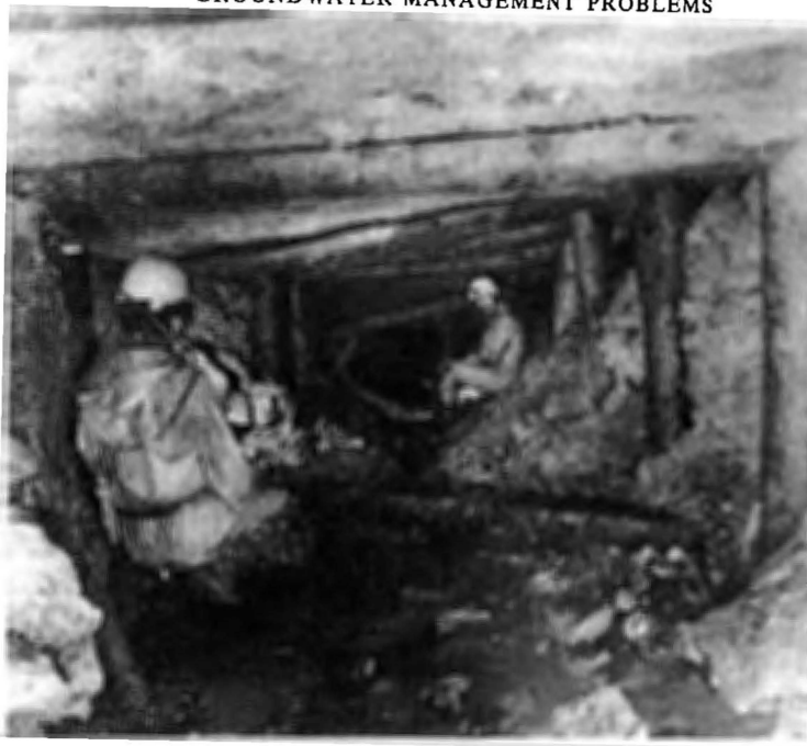
FIG. 7. Free drainage in mine workings abandoned in 1956. Closure of the adjacent mined galleries by swelling of the seat earth has occurred, and the stone retaining walls on both sides of the roadway have collapsed. Seat earth is being eroded by the small stream keeping the roadway open, below the intact Pennant Sandstone roof.
